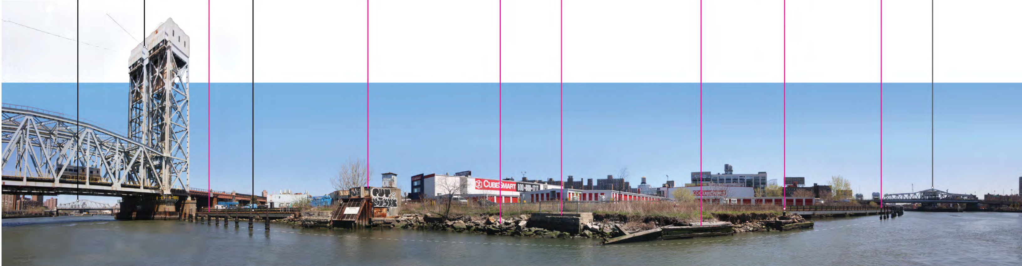
Metro North Bridge
